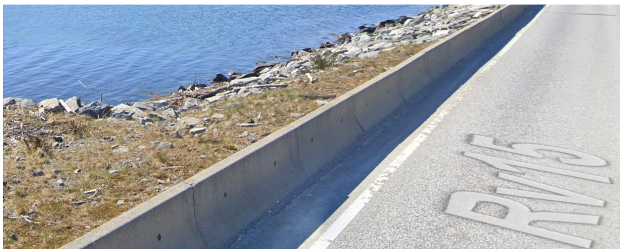
Figur 2-4: Betongkant langs rv.15.
